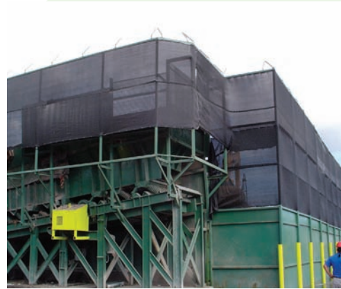
Fine Mesh Screen Dust Control Placed Over The Pollutant Source
